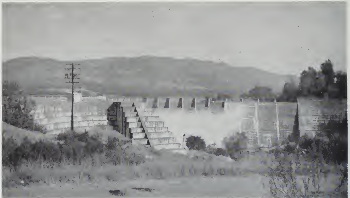
Hogan Dam on Calaveras River
